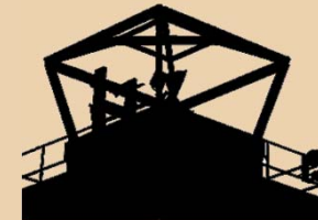
Control tower from original factory remains on the building
