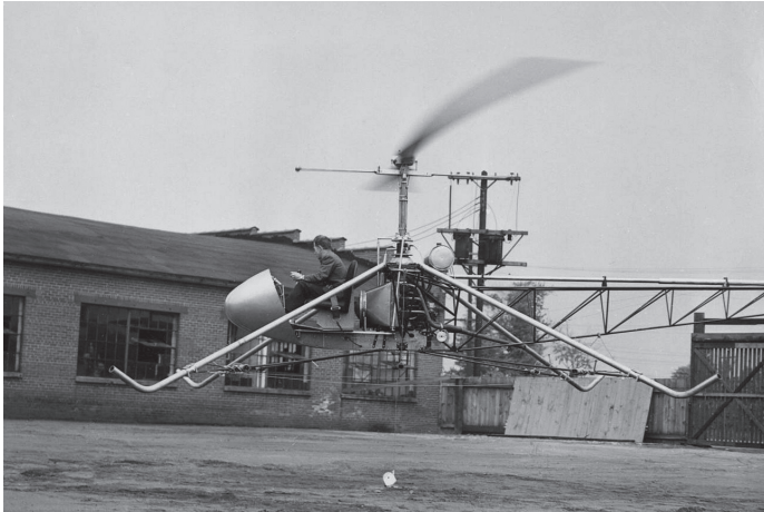
The first helicopter was named Lady Genevieve. Here it is in a tethered hover being flown by Arthur Young. Once controllability was verified, the outriggers were removed and a wheeled landing gear installed, along with an outer shell on the sides of the cockpit and around the engine compartment and tail boom.
